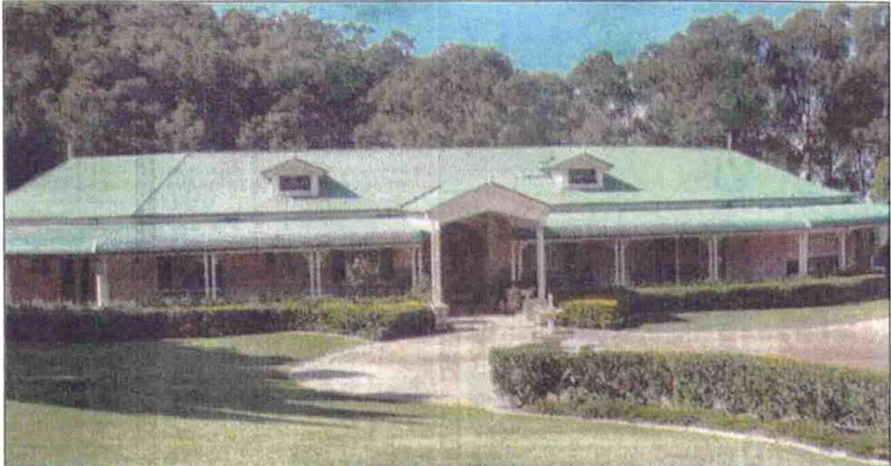
BOOMING ESTATE: The Glasshouse Mountains Estate is taking off with homes being constructed on site
